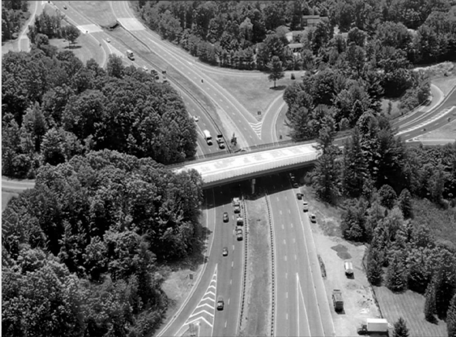
Weldon Road over Route 15 Emergency Bridge Replacement Jefferson Township, New Jersey
